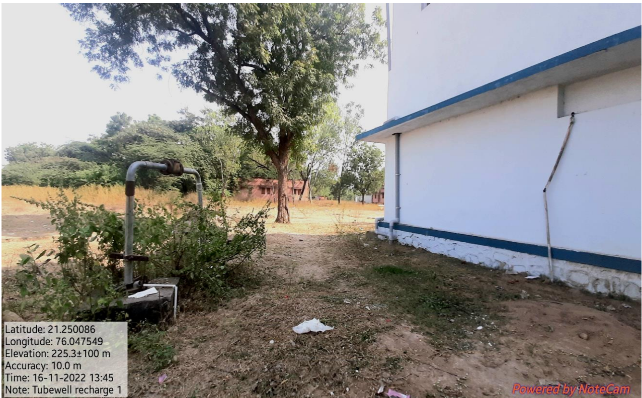
Bore Well Recharge by Rain Water and Roof water
