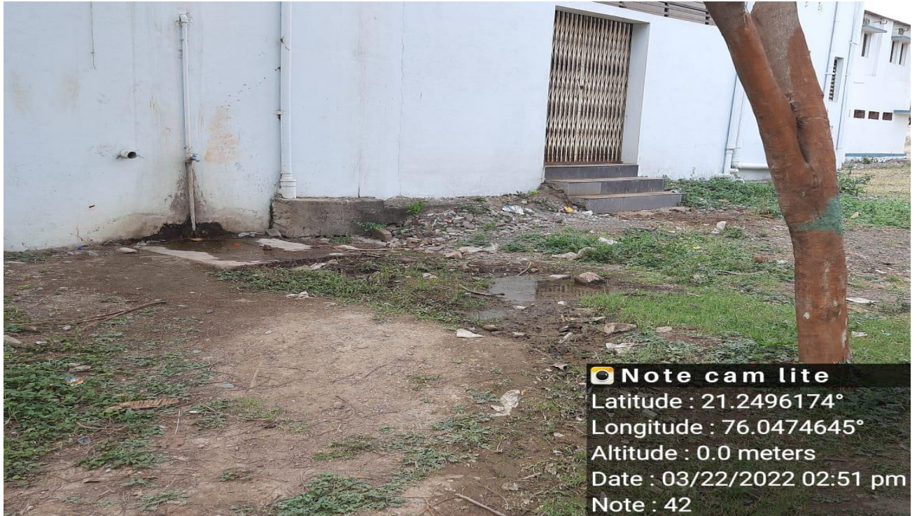
Waste Water Used for Gardening
