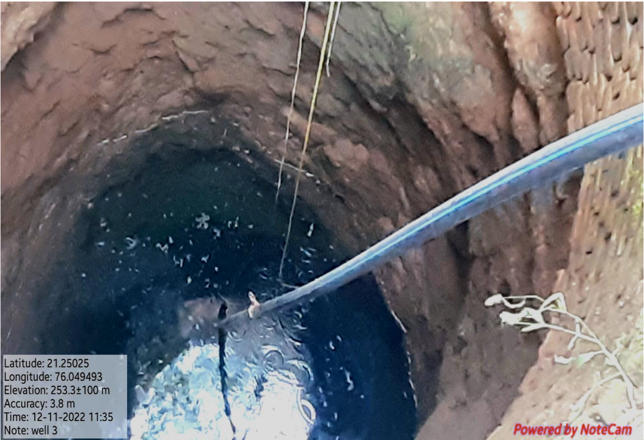
Open Well Recharge by Rain Water
