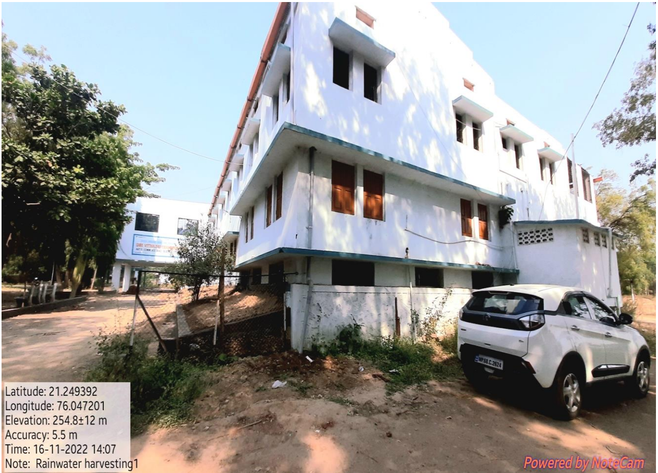
Rain Water Harvesting
